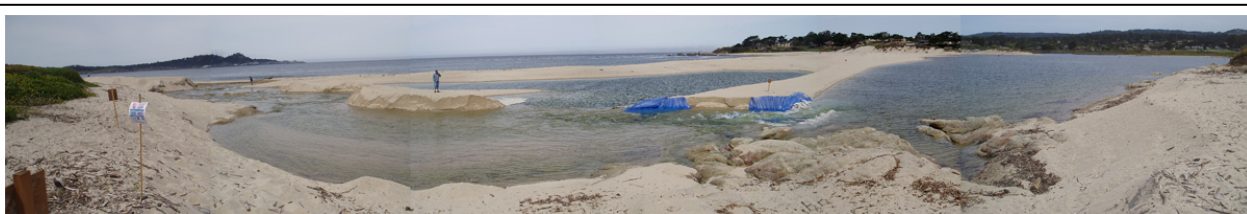
Temporary sandbags and tarps were used to raise the lagoon water level in Summer 2006
