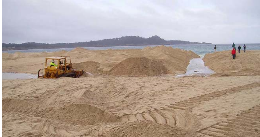
Cutting an outlet through the beach - December 2004
