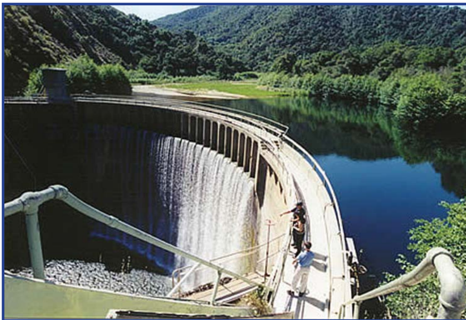
San Clemente Dam
