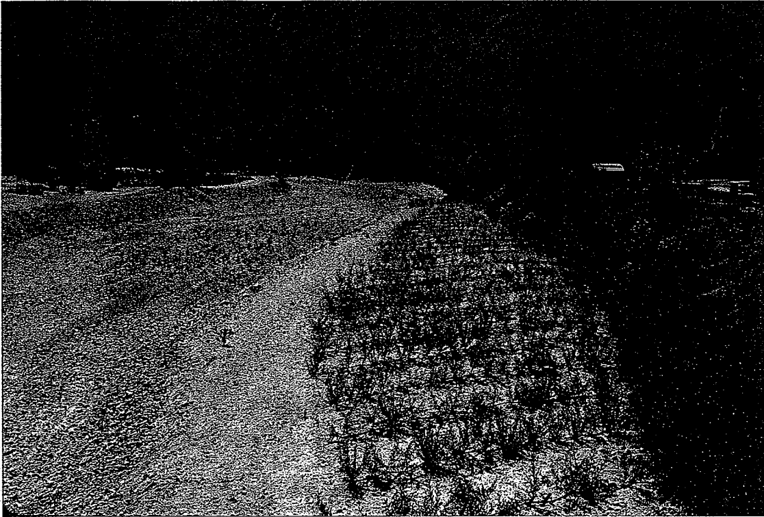
Picture 3 (late-1980's) from the same location as picture 2: shows how user fee funds were used to restore the bank by reshaping the channel and planting riparian vegetation on the bank. These trees have been irrigated to offset water extraction (note the dry river bed)
