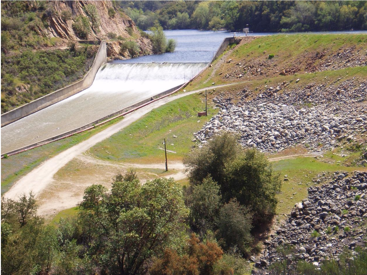
Los Padres Dam – looking upstream at dam and spillway
