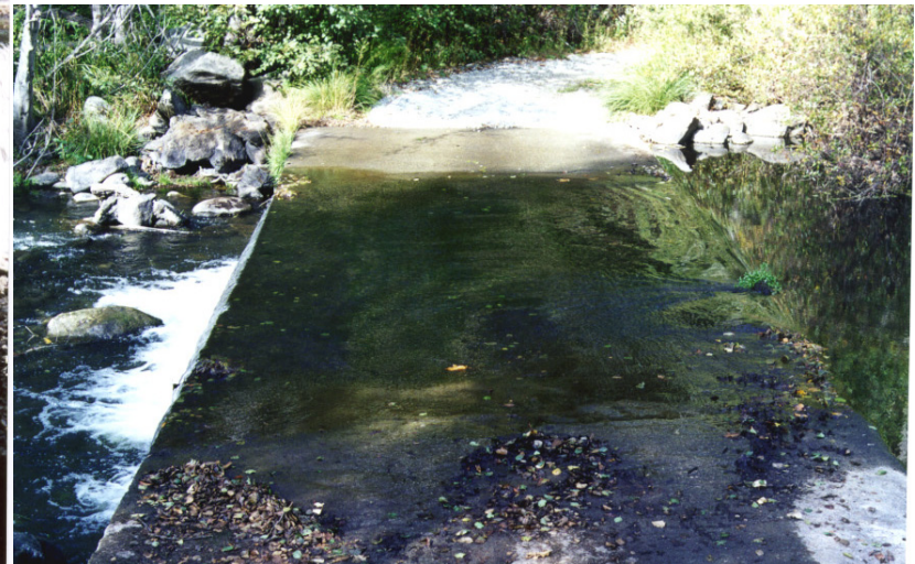
Looking north from center of ford toward approach
