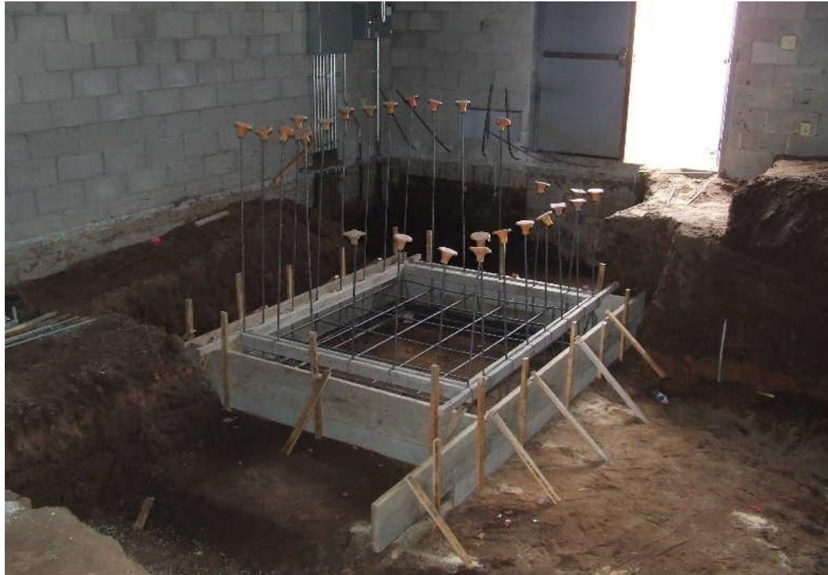
Subfloor pit installation in control room
