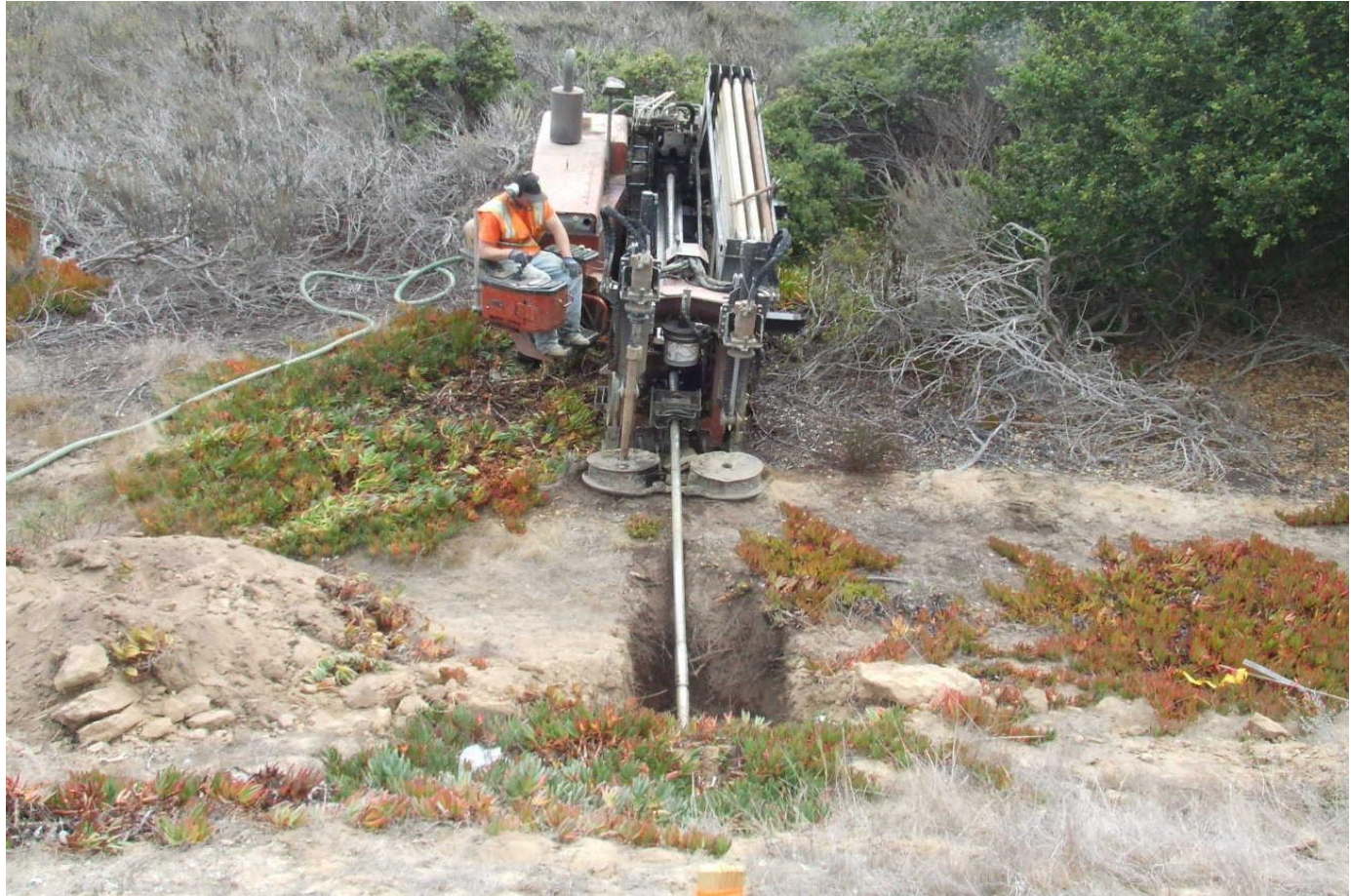
Directional drilling under roadway
