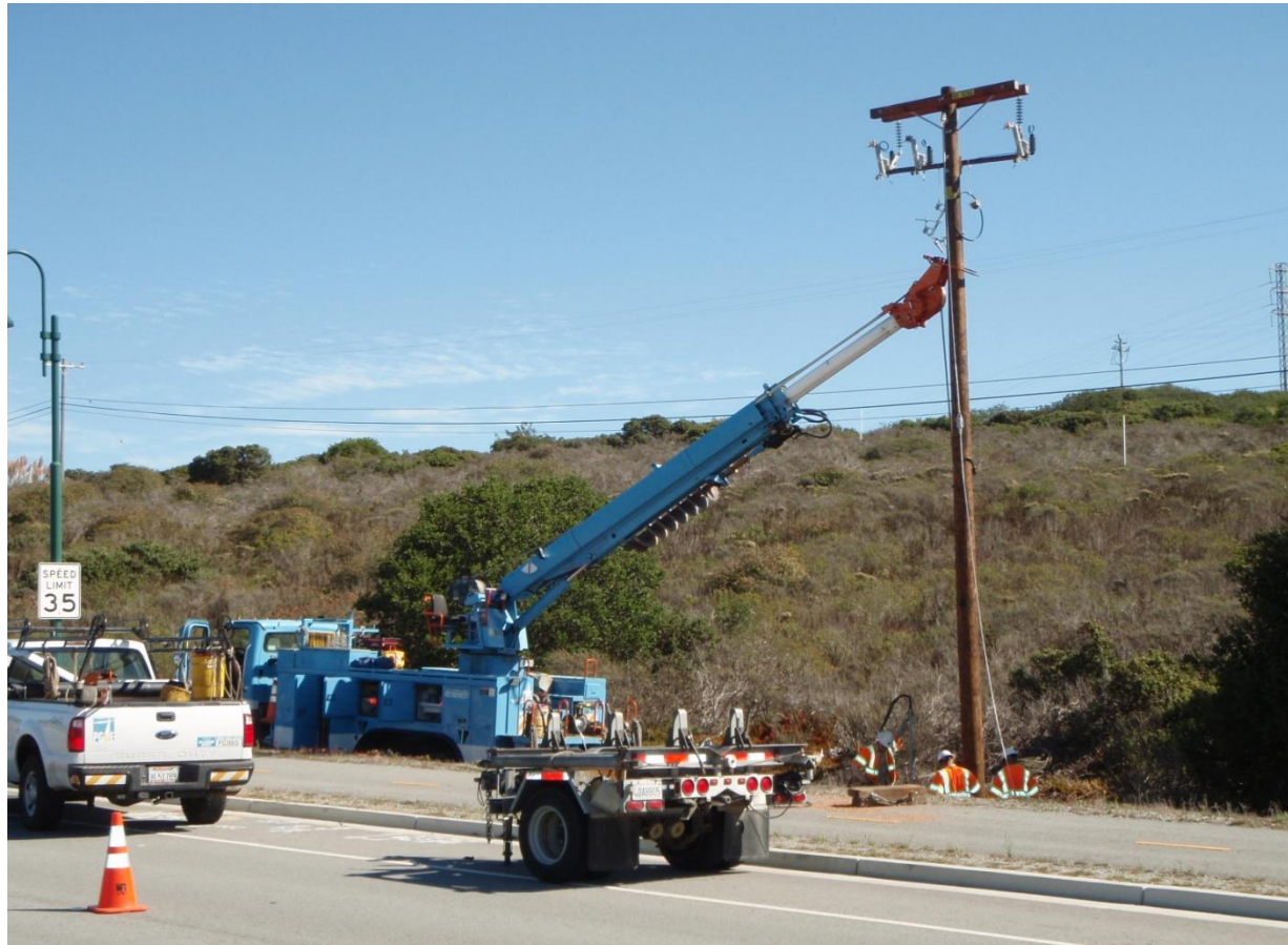
PG&E crew extending power service to site
