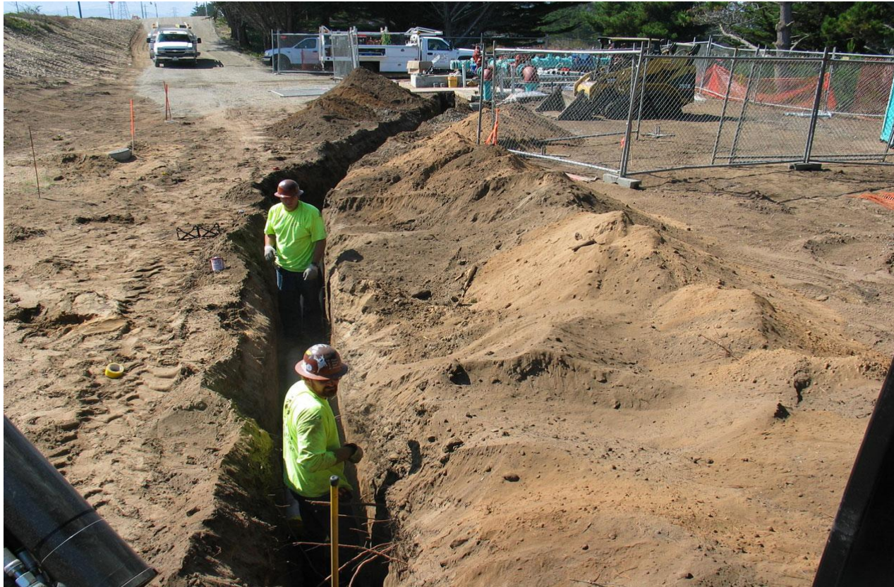
Trenching for electrical conduits
