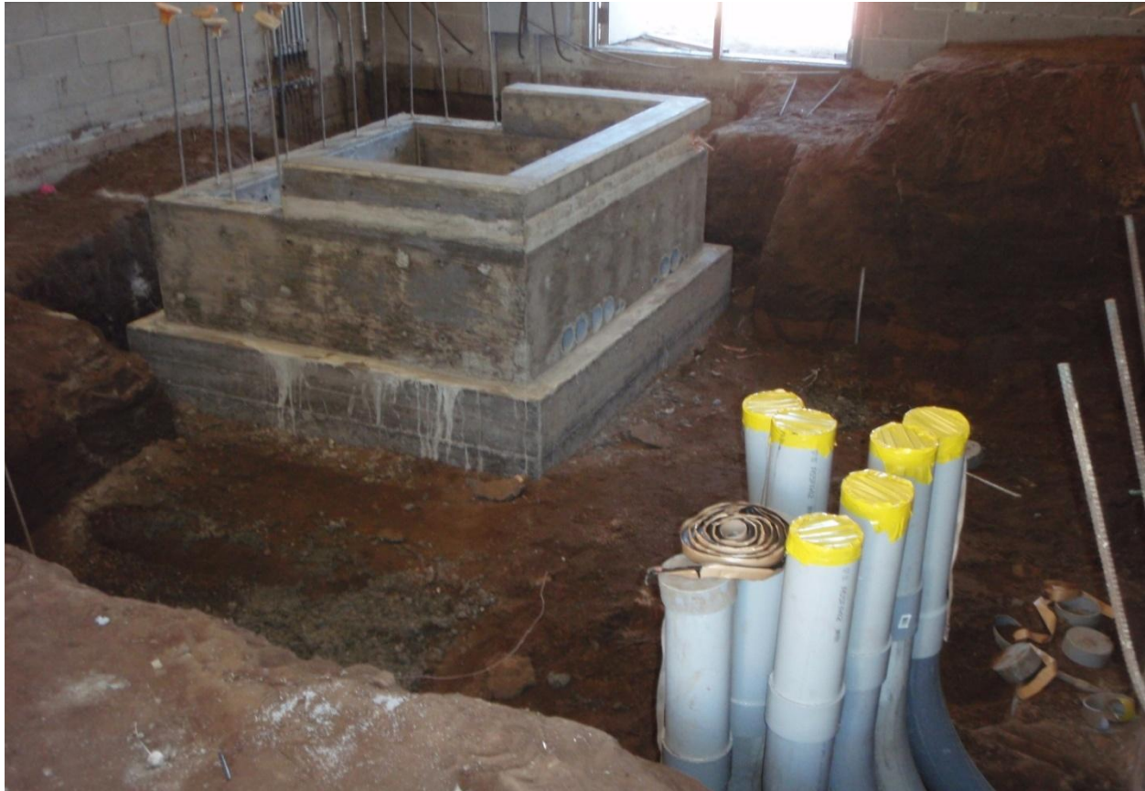
Electrical conduit installation in control room
