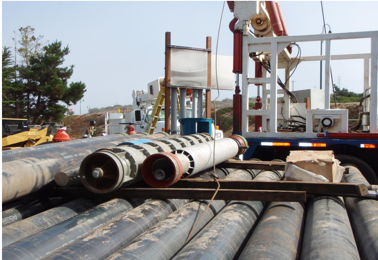
Pump and flow control valve installation
