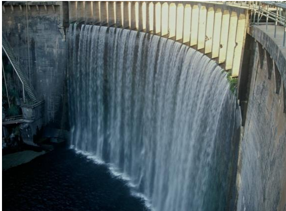
San Clemente Dam
