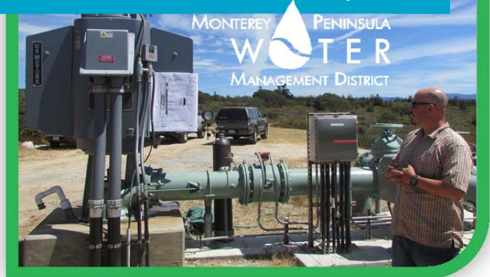
Water District's Aquifer Storage and Recovery project site.
