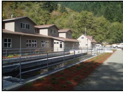
Four refurbished raceways in front of the OHRC building
