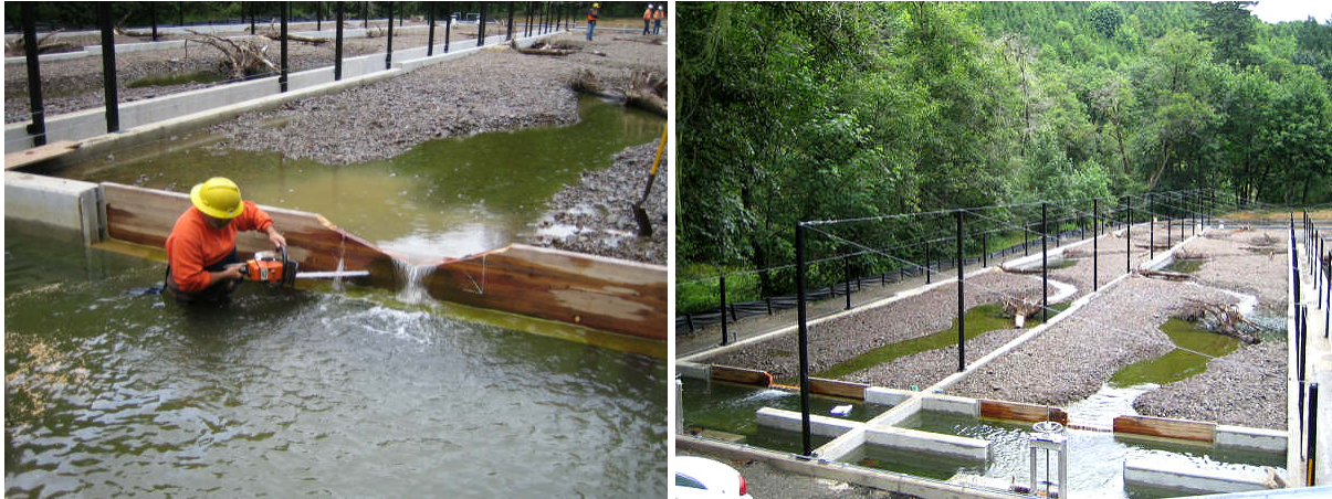
A mixture of river gravels and woody debris was placed to provide improved habitat. Shade cloth suspended above the streams simulates tree cover.
