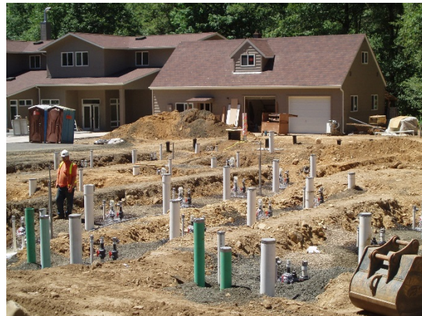
The new research building is 18,000 sf, including wet lab, quarantine lab (with effluent disinfection) and dry lab facilities. A 10,000 square foot tank farm area is located adjacent to the new research building. (Underground piping system is shown under construction at right.)
