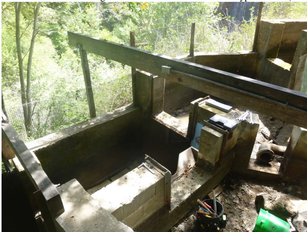
SCD Ladder after decommissioning of fish counter and downstream bypass chute (2015).
