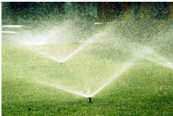
High Use Inefficient Fixed Spray Sprinklers
