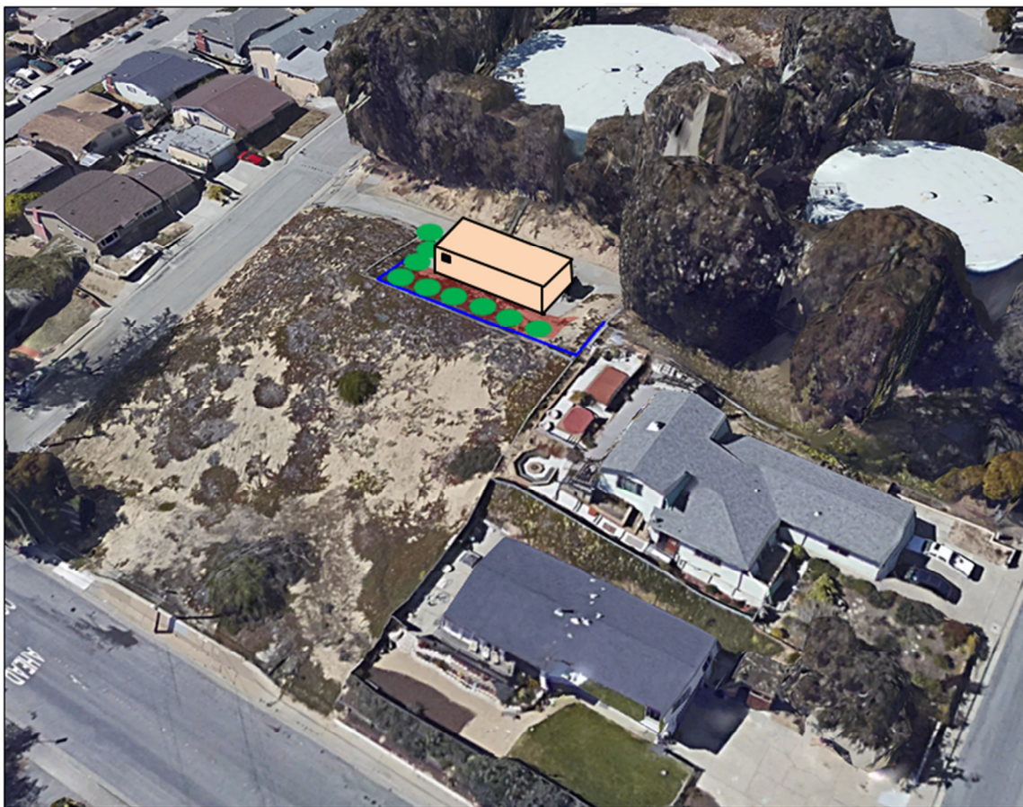
Figure 1. Aerial view of Project vicinity and proposed conceptual pump station enclosure (not to scale)
