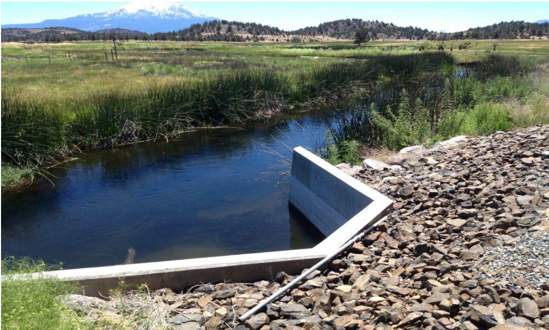
Image 1- Example of alcove built into stream bank to house a cone-shaped fish screen.
