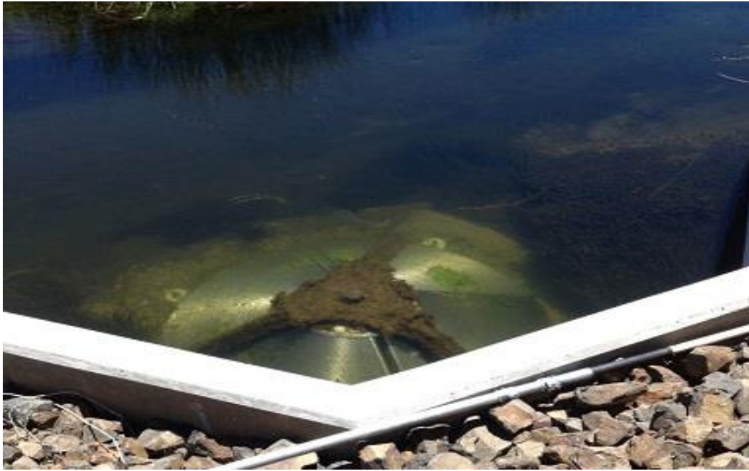
Image 2- Example of cone screen underwater in an alcove with external cleaning brushes in operation.
