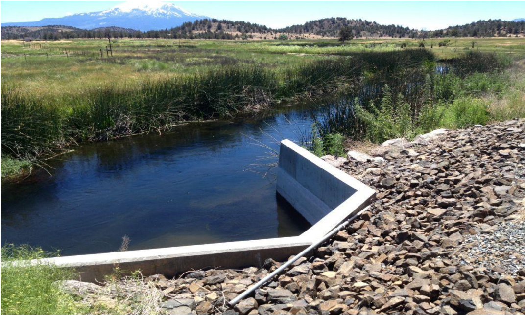
Image 1- Example of alcove built into stream bank to house a cone-shaped fish screen.
