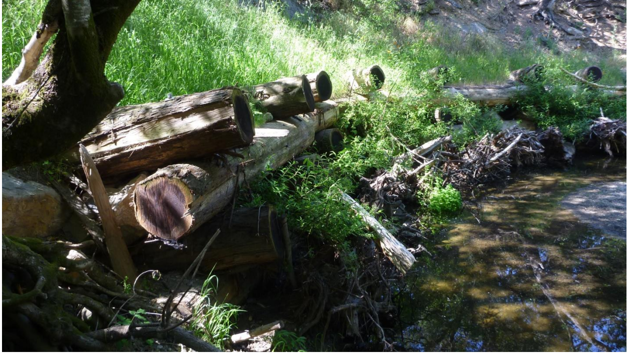
Figure 6. Example of completed log cribwall
