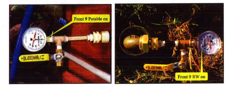
Following confirmation that all outlets on both systems were confirmed to be on, the potable system was shutdown at the potable RP service at 1420. Once the potable system was shutdown and and the RW system remained pressurized all outlets on both systems were checked for pressure/flow. It was then confirmed that only the potable outlets were off at this part of the test. See pressure gauge images below.
