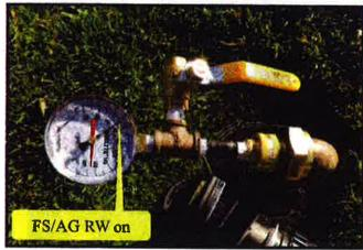
Following confirmation that shutting down the potable services did not impact any RW outlets, the potable services were restored at both potable RPs. The RW system in both areas were then shut down at 1100. It was then confirmed that only the RW outlets were off and the potable system remained pressurized at this part of the test. This took place at 1300. See pressure gauge images below. No cross connections were discover in this area.
