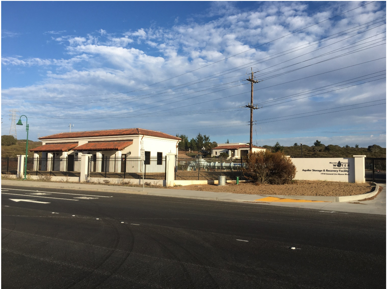
(Photo: Aquifer Storage & Recovery Treatment Facility)
