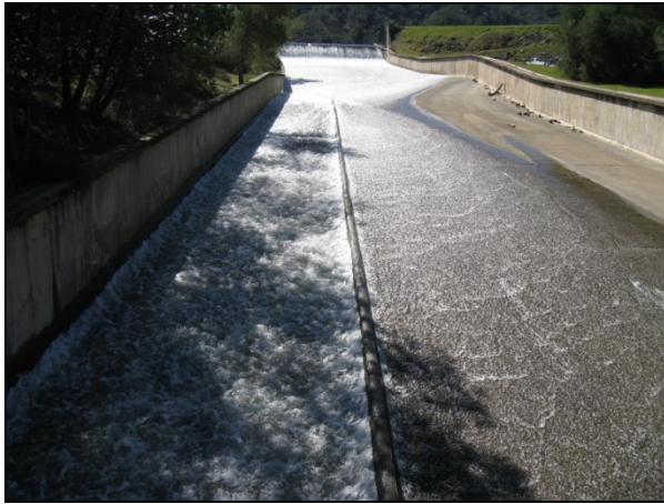
Photograph 3. Spillway with concrete berm oriented on the left hand side of the photograph.
