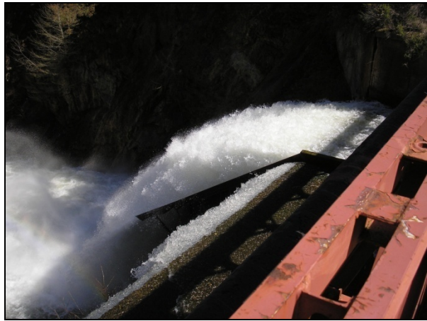
Photograph 4. Steel ramp attached to spillway outfall.
