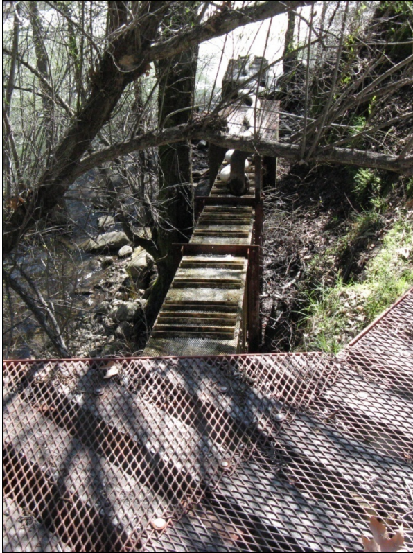
Photograph 5. Denil type fish ladder, auxiliary water supply pipe (center), and adult fish trap (foreground).
