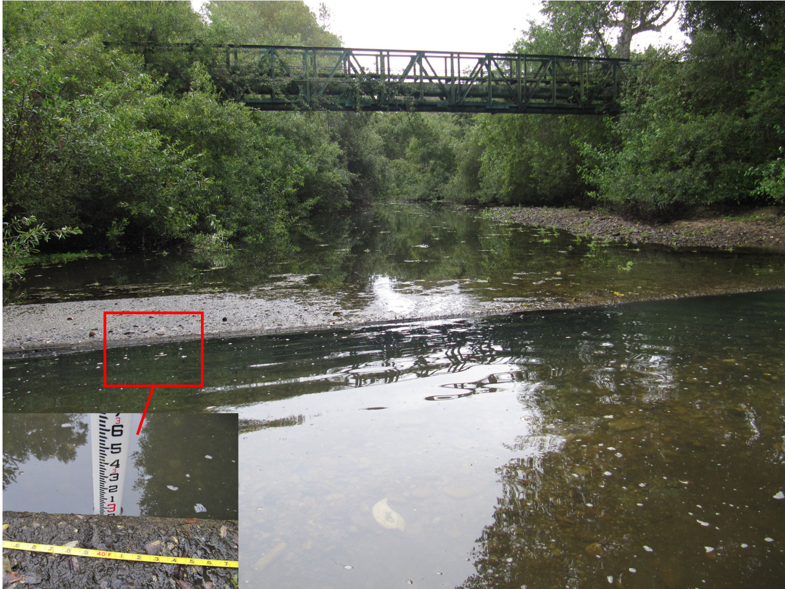
Figure X-2 – Carmel Area Wastewater District Pipe Crossing (looking upstream)
