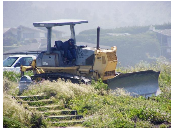
Flood Control Work –Carmel River Estuary
