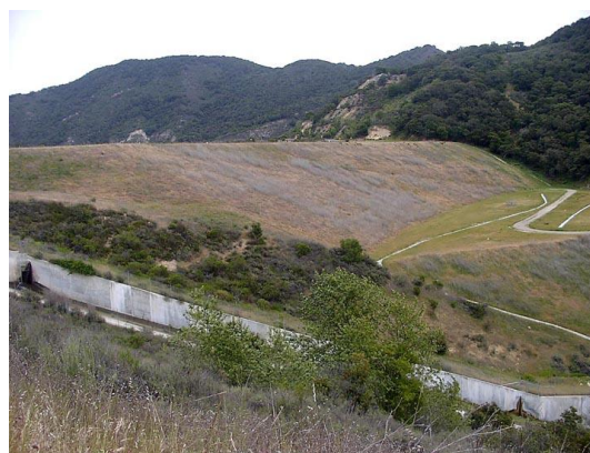
Lopez Dam – Arroyo Grande Creek
