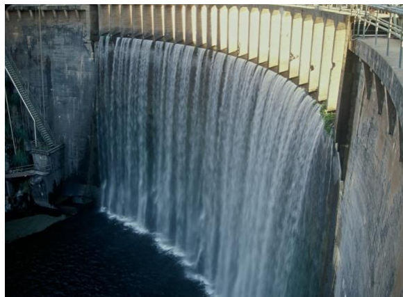
San Clemente Dam
