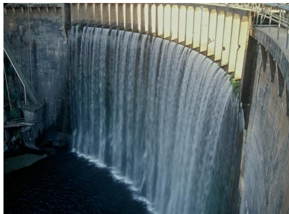
San Clemente Dam
