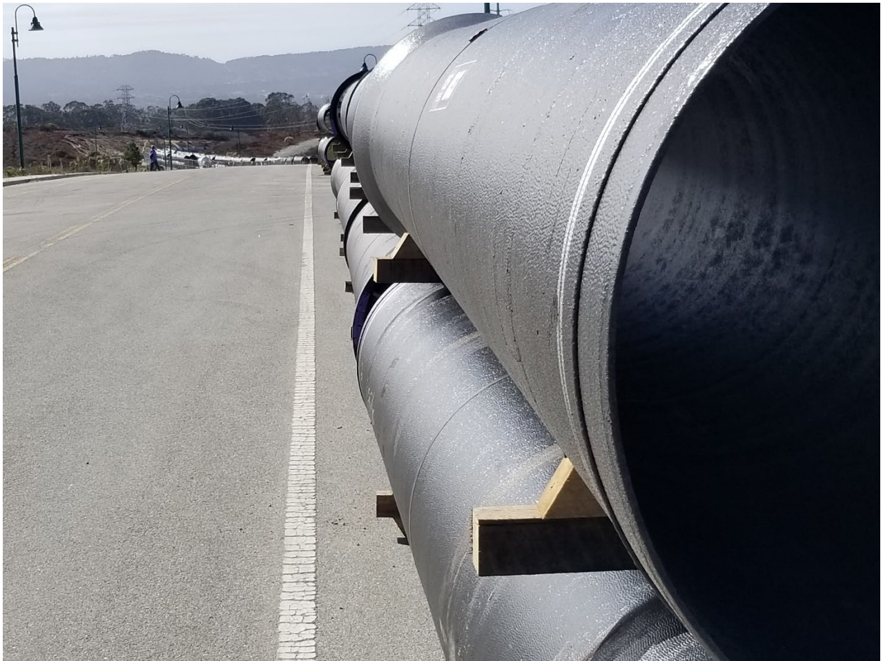
(Photo: Gen Jim Moore Blvd Pipe Installation)
