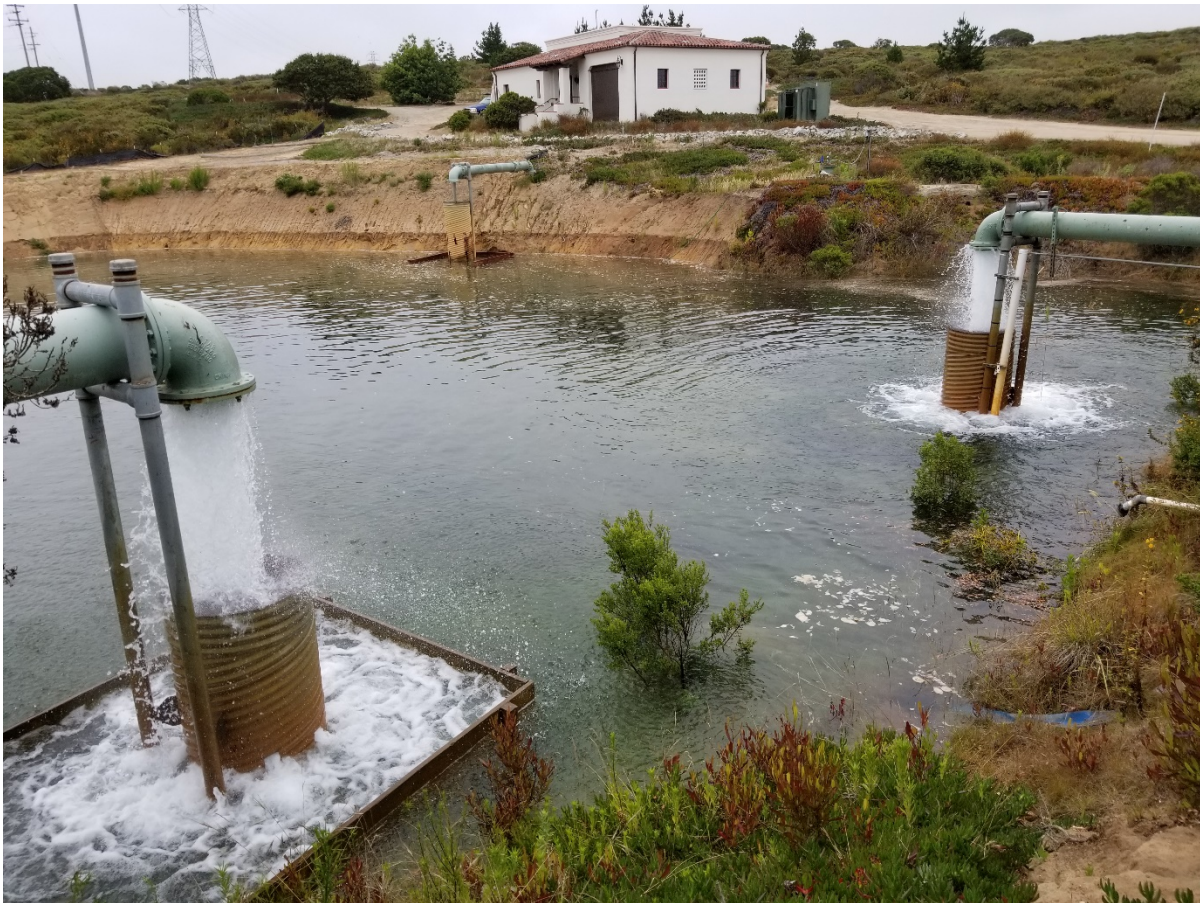
(Photo: Aquifer Storage and Recovery Backflush Basin)
