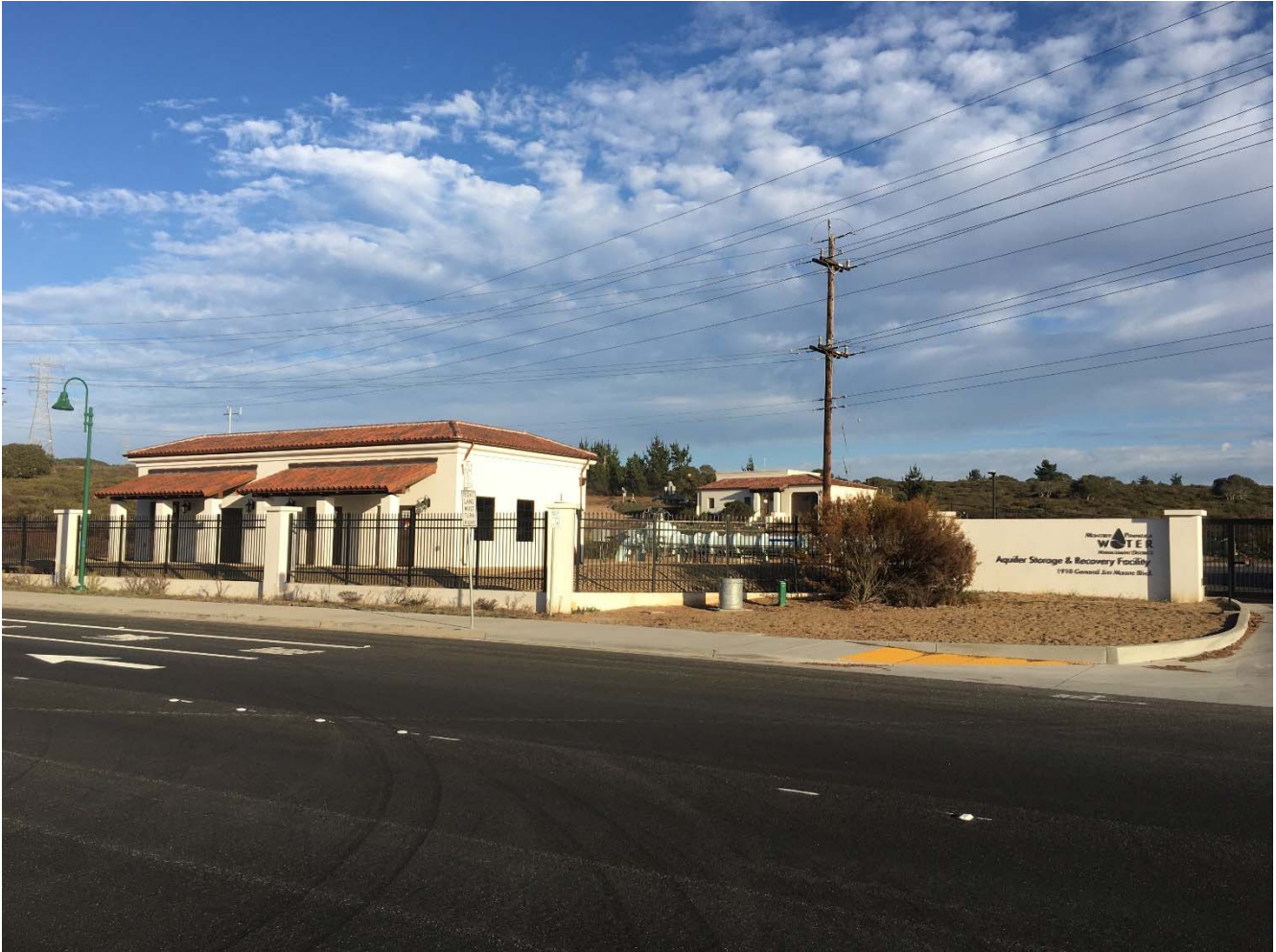
(Photo: Aquifer Storage & Recovery Treatment Facility)
